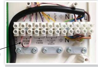
FIGURE 21. ELECTRICAL CONNECTIONS
